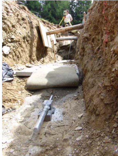
Figure 4: Sensor S2 whilst embedding
